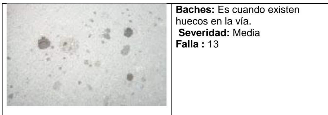
Falla baches (Autor, 2015)
